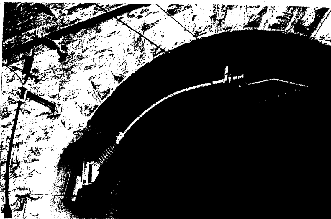
Figure 4: Tunnel catenary support structure with silicone composite insulator in a single track tunnel of the BN Bern - Neuenburg line. At the extreme left a 30 kV silicone cable sealing end can be seen.
