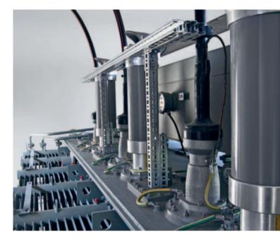
HV CONNEX surge arrestors installed in a power transformer.
