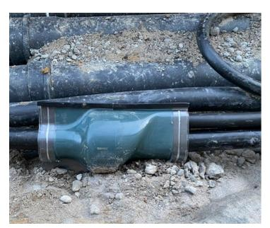
Cable branch using AM130/300 cast resin joint filled with FILLBRH
