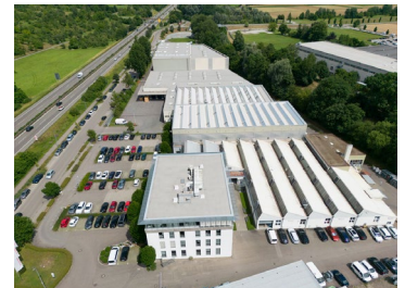
PFISTERER Group headquarters in Winterbach, Germany
