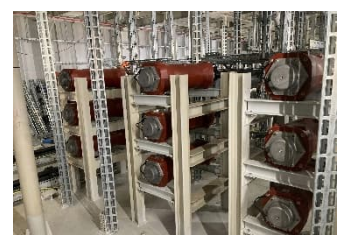
For power transmission that is safe in the long term, PFISTERER installed around 200 CONNEX inner cone connectors, epoxy resin joints and link boxes.
